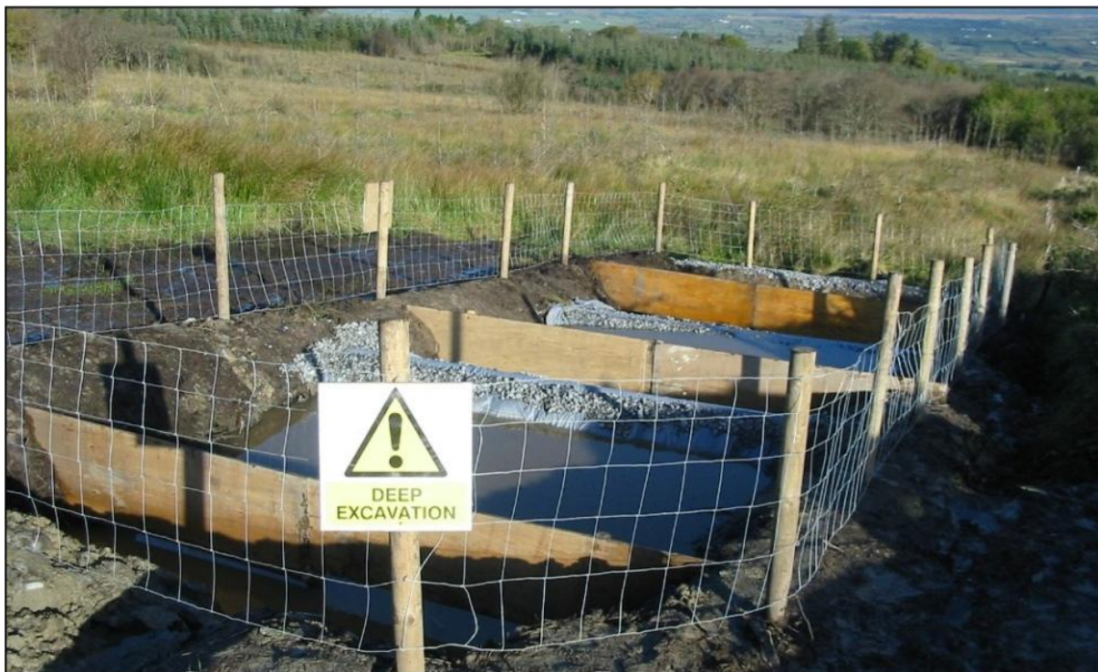
Figure 4-3: Typical Three-tiered Settlement Pond with Stone Filter
